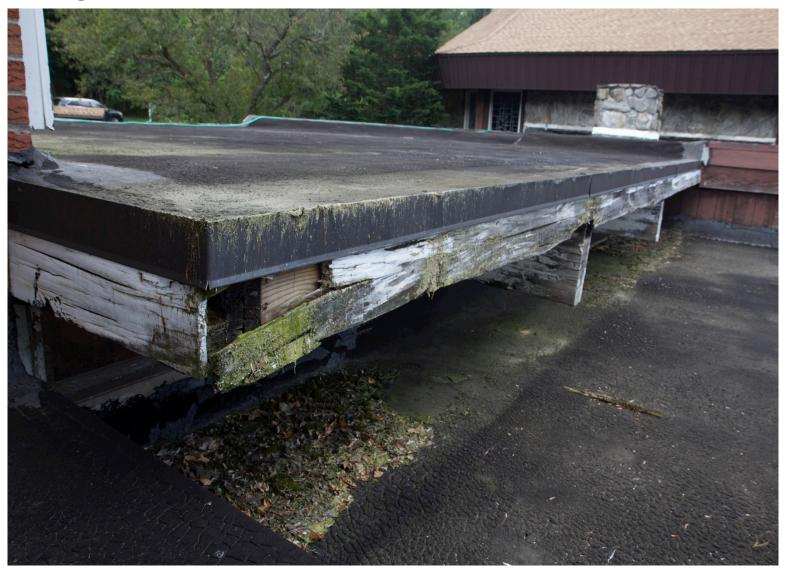
• Rainwater pools and sits. When the rain drains, it drains through the roof.
